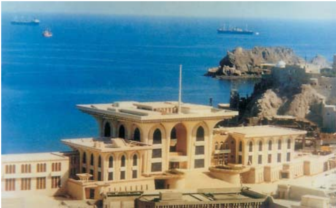
The Palace of His Majesty Sultan of Oman, Muscat, constructed by Shapoorji Pallonji & Co. Ltd.
